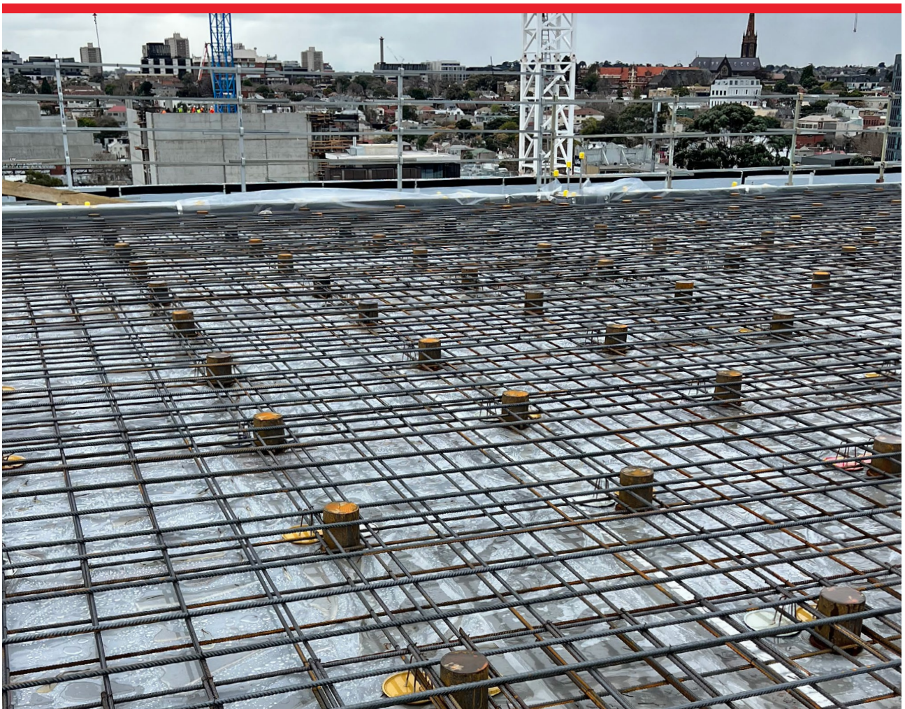
FS Jack up mounts installed prior to concreting.
