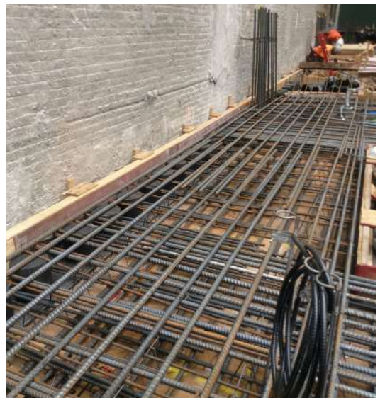
Transfer slab reinforcement installed and slab poured
