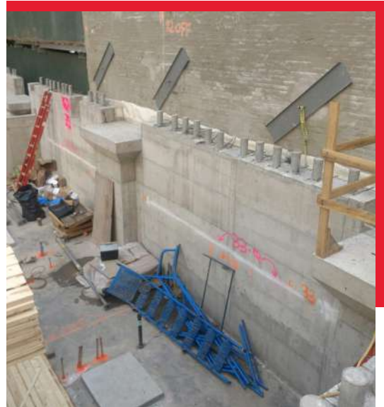
Wall is formed and shear pin is core filled
