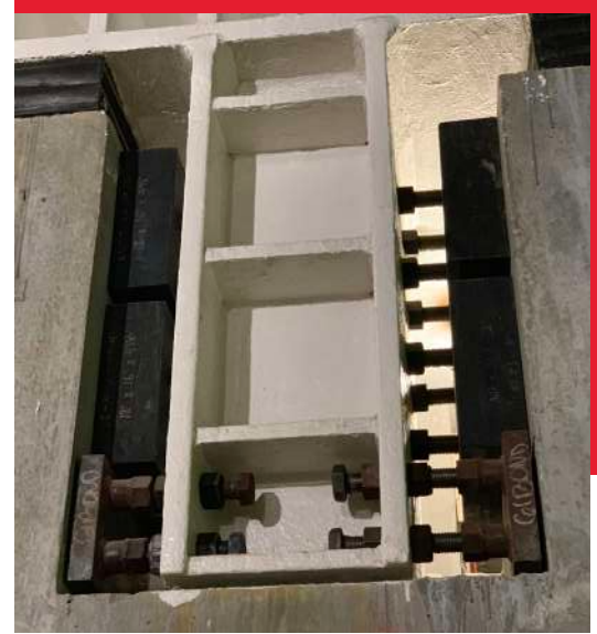
Lateral bearings pre-loaded with overload stops
