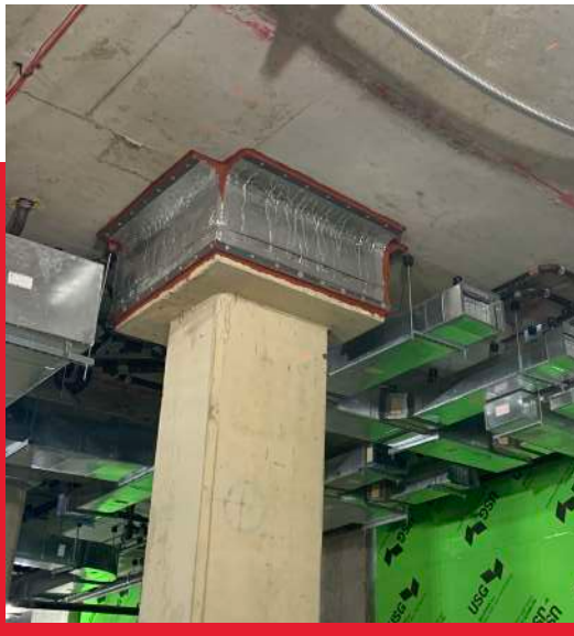
High load bearings at column capital with Fire Proofing installed
