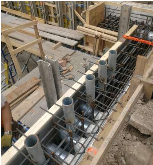
Shear pins are tied off to shear wall formwork
