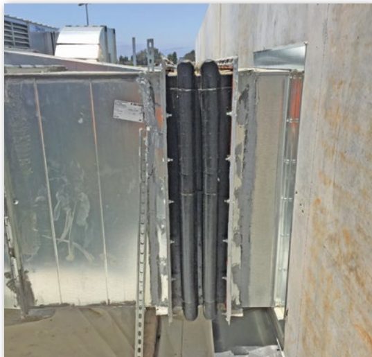
ME-2, 2 Arch Rectangular Duct Connector installed.
