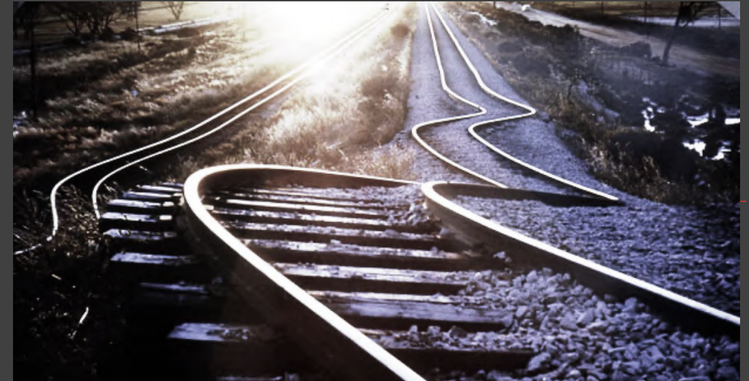
Railway line deformed by magnitude 6.8 – Meckering WA - 1968
