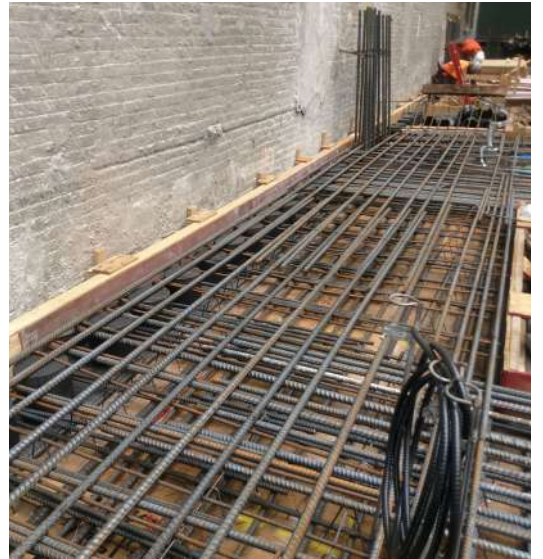
/ Transfer slab reinforcement installed and slab poured
