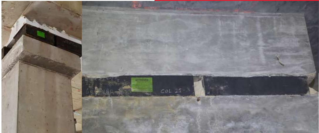
High load bearings at column capital with shear pins within bearing array
