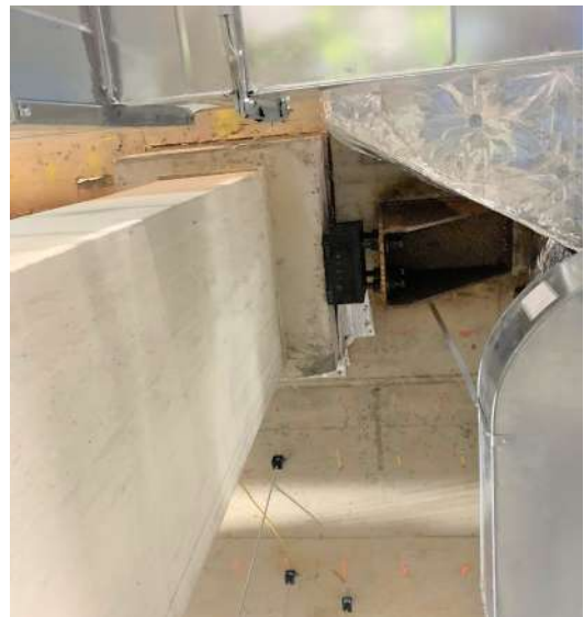
/ Lateral Restraint Blocks at walking columns
