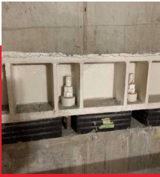
/ Isolated tension restraints installed within shear key
