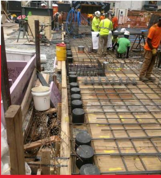
/ Shear key caps and bearings installed on top of shear wall. Sand packed to height of bearings
