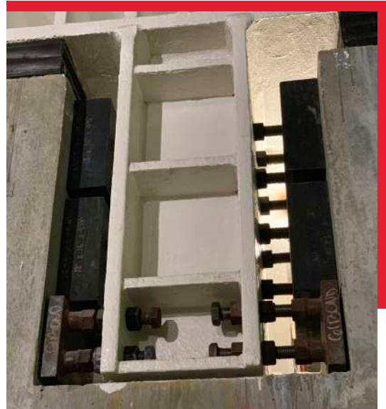
/ Lateral bearings pre-loaded with overload stops
