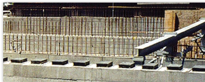
Leveled Isolation Pads Resting on Foundation Wall Prior to Continuing Construction
