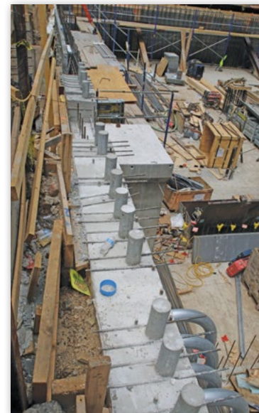
Isolated Shear Pin Pipes cast into perimeter wall in Manhattan
