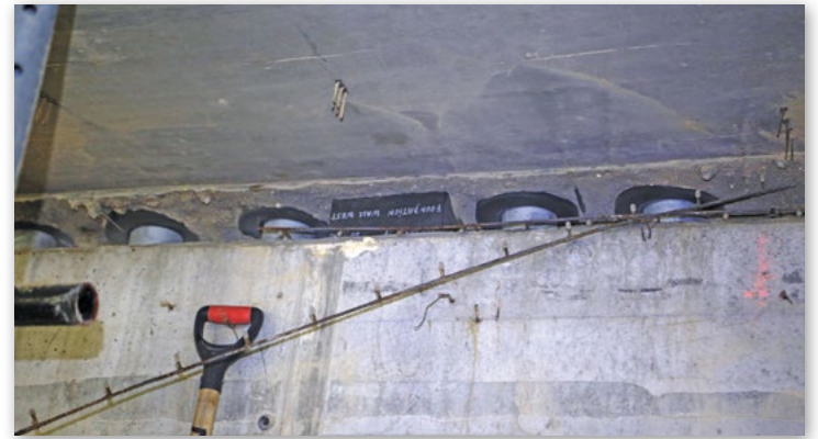
Isolated Shear Pins cast into the perimeter wall of a building in Manhattan
