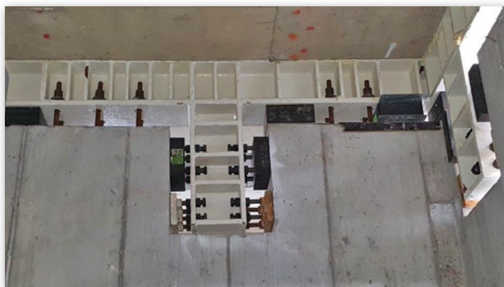
Perpendicular Isolated Shear Keys in a Brooklyn Hotel
